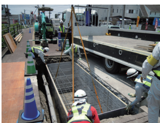
②型枠設置
