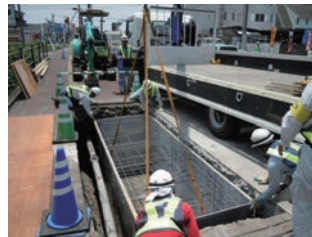
②型枠設置
