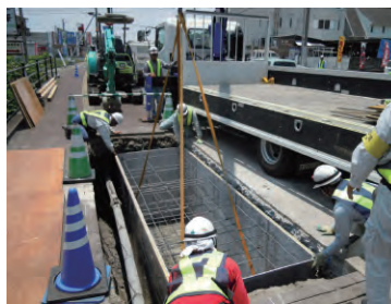
②型枠設置
