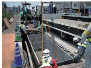
②型枠設置
