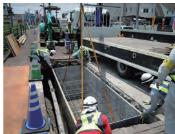
②型枠設置
