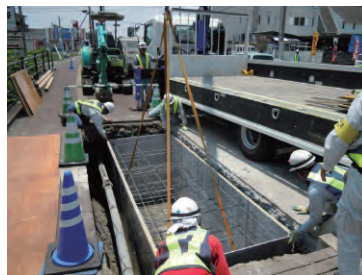
②型枠設置
