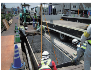
②型枠設置
