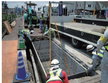
②型枠設置
