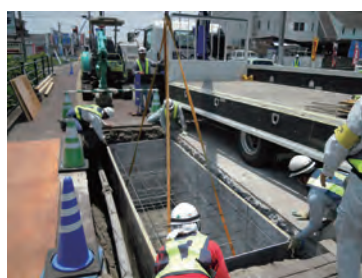
②型枠設置
