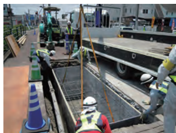
②型枠設置
