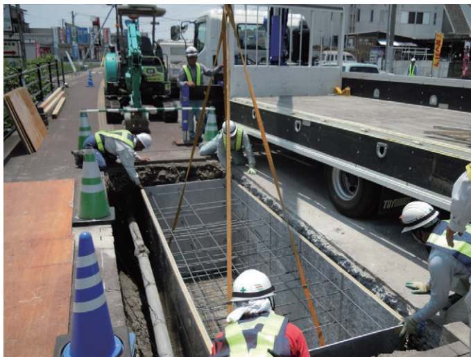
②型枠設置
